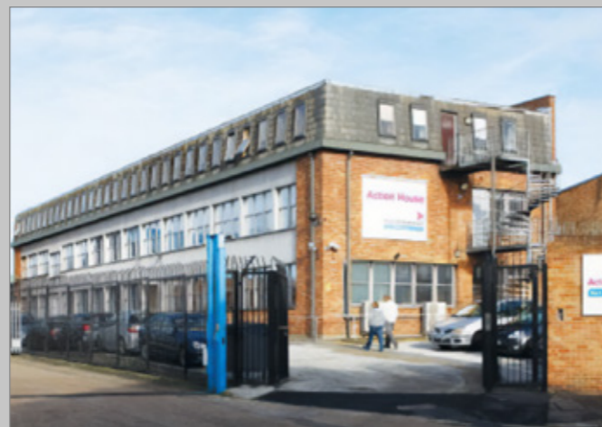
53 Sandgate Street (Site 1)
